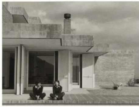
Photographs taken at Casa Coderch, Sant Feliu de Codines. Architect: José Antonio Coderch
