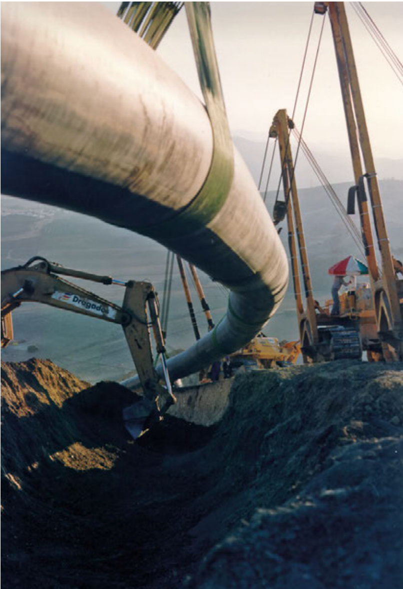
Construction work on the Maghreb-Europe gas pipeline, 1996. Archive Naturgy.
